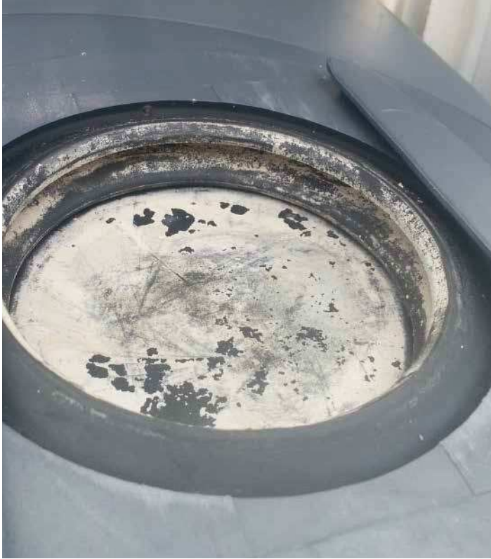
An old lip seal in need of replacement.
