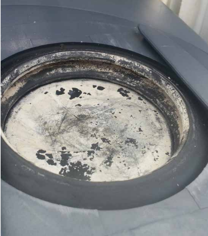
An old lip seal in need of replacement.
